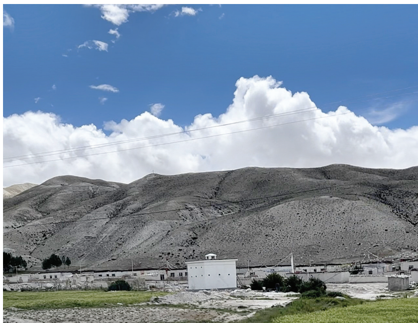
Figure 17: Newly built Mang Gang at Namashung
