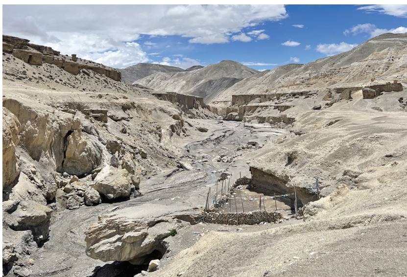
Figure 3: Lhae or Chhuprang, a traditional structure of keeping goats, near drying river
